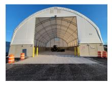
Road salt being delivered into DPW's new salt storage building. This new building will reduce downtime for plow drivers not having salt chunks in the spreaders anymore and reduce cost from the weather not being able to run off the pile anymore.
