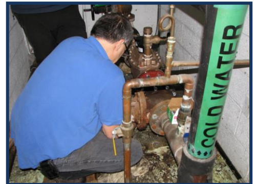
New Meter in Place
