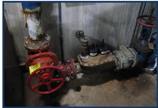
New Meter and Valve In Place
