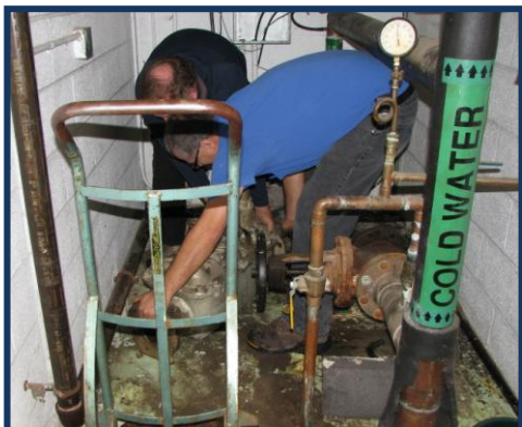
Removing the Old Meter
